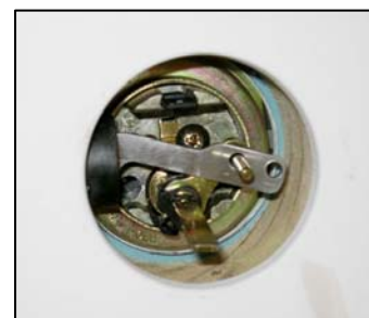
Photo 15 Actuator pin is shown in the 2 3/8" backset hole
