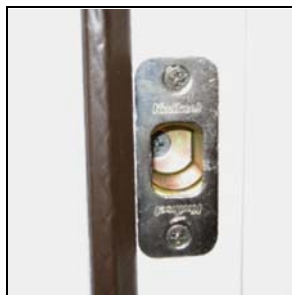
Photo 2a Dust plug inside deadbolt strike plate
